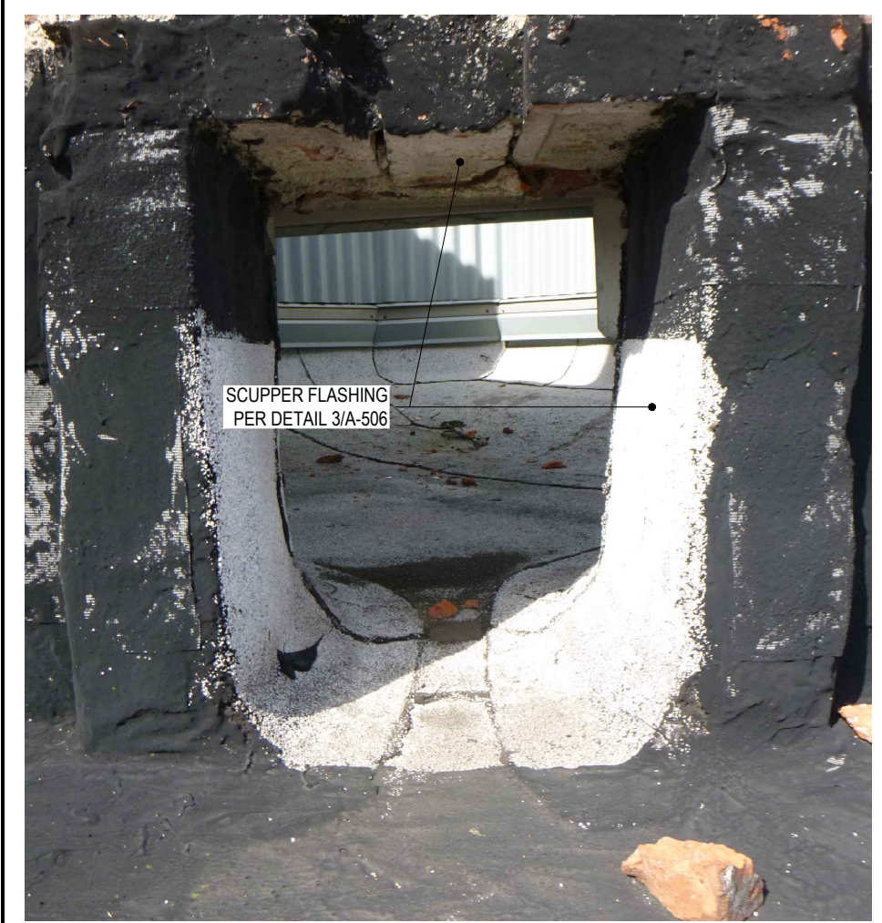
6 SMALL TURRET SCUPPER REF: 5/A-508 SCALE: NTS
