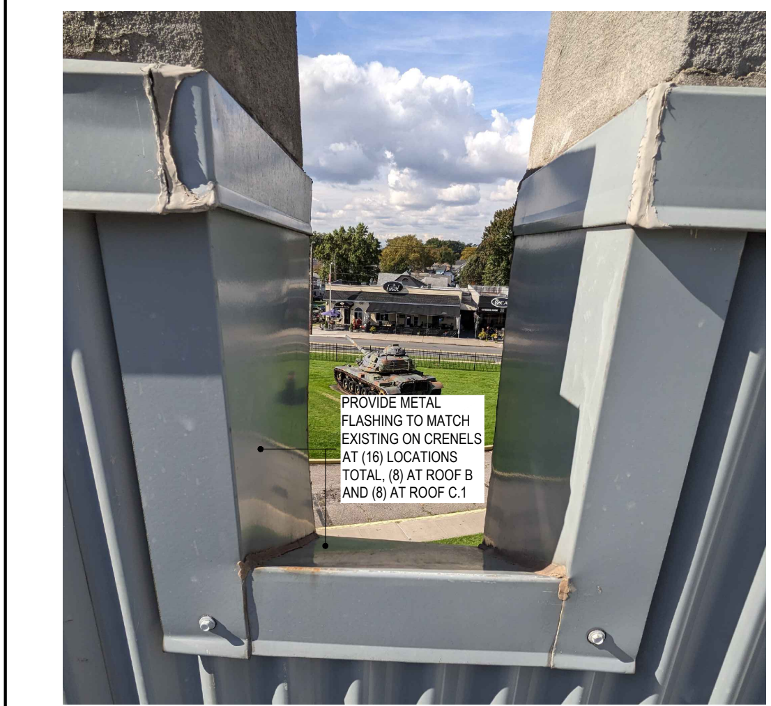
8 CRENEL FLASHING REF: SCALE: NTS
