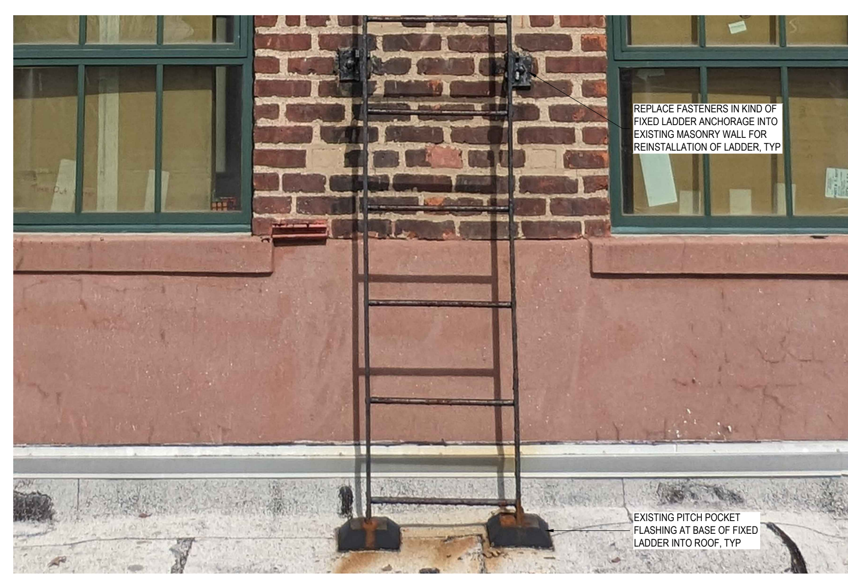
3 EXISTING FIXED LADDER REF: 1/A-507 SCALE: NTS
