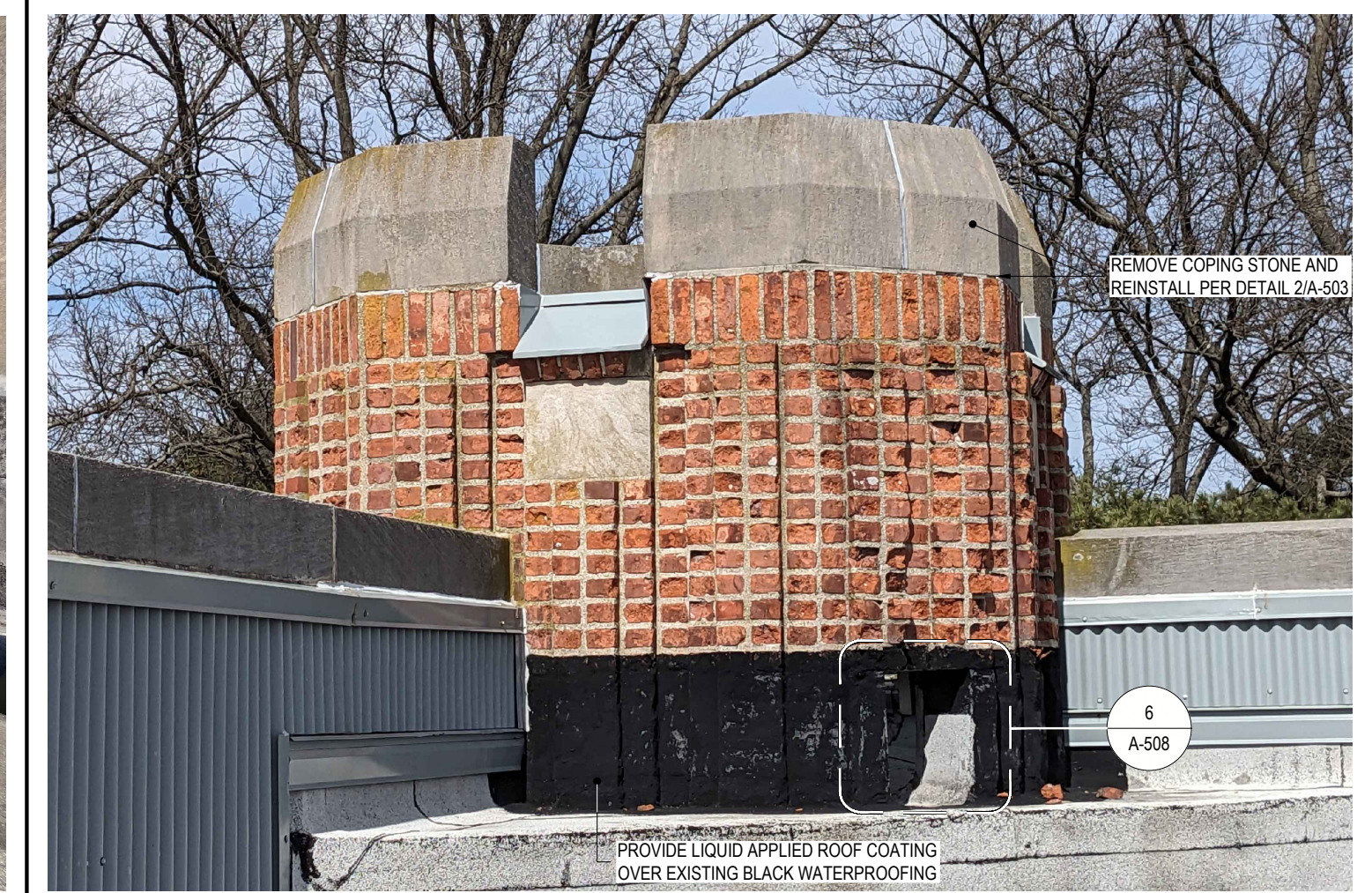
5 SMALL TURRET SCUPPER LOCATION REF: SCALE: NTS
